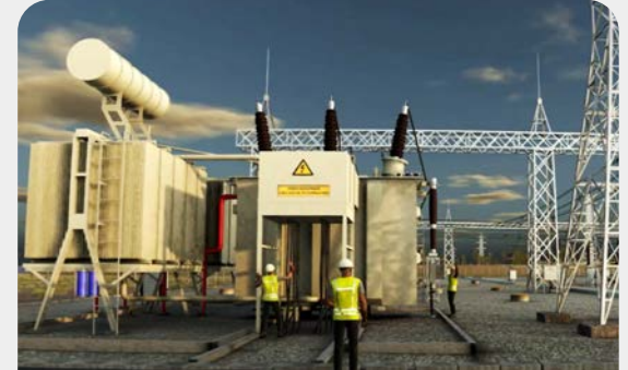
Project: Maintenance of Power transformer (360 VR) Clients: Evren
