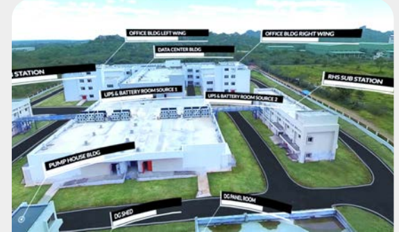
Project: Data center technical walkthrough (multi format) Client: KEC International
